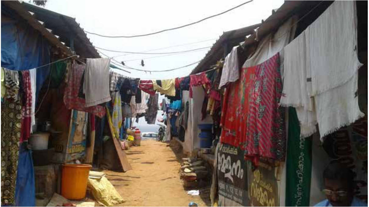
Fig 4.3 Improper and Congested Rehabilitation Units in Mathipuram Colony .
